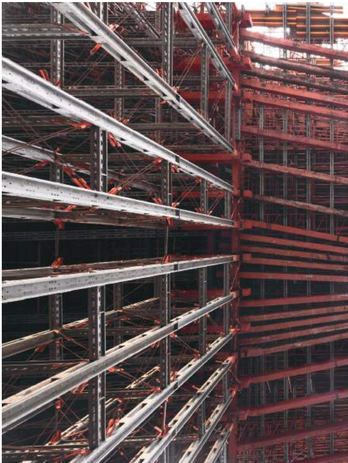
Landscape Under Construction Alfonso Batalla
