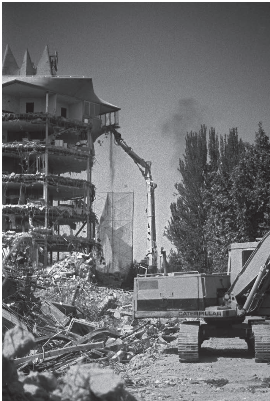
Demolition of Miguel Fisac's La Pagoda. Madrid, 1999
